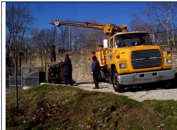
Figure 5: Maintenance of floatables nets at T-04
