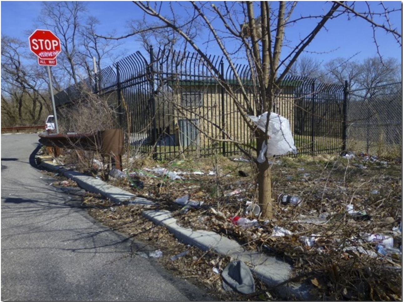
This next photo shows an unscreened drainage channel to the left of the building when facing the front doors.
