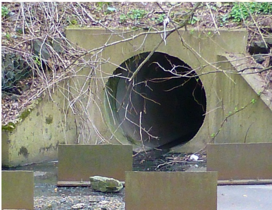
A. Outfall and concrete channel
