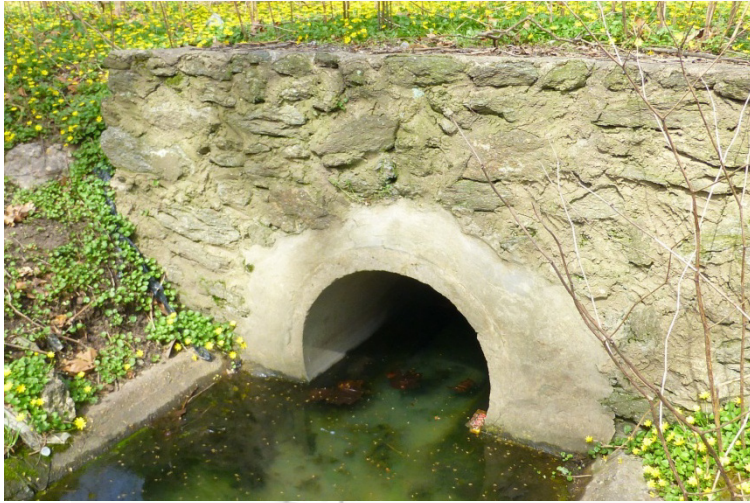
A. Outfall and concrete channel
